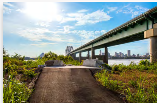
Big River Crossing project, Memphis, TN
